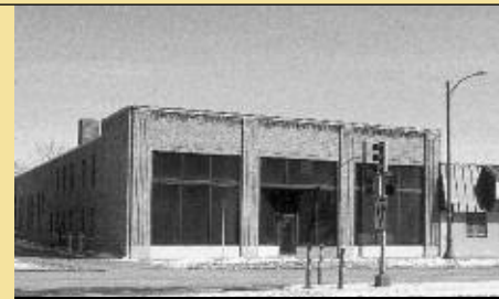
NCC First Building (after)
